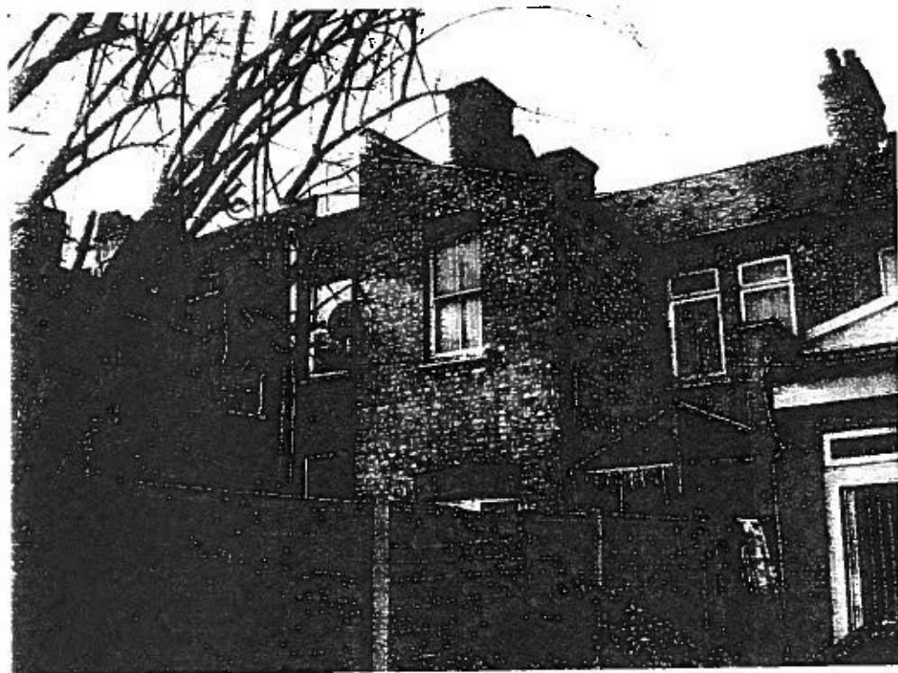
View south along the rear of the terrace
