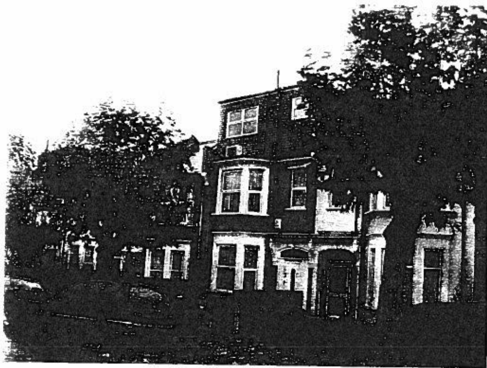
View north along the street
