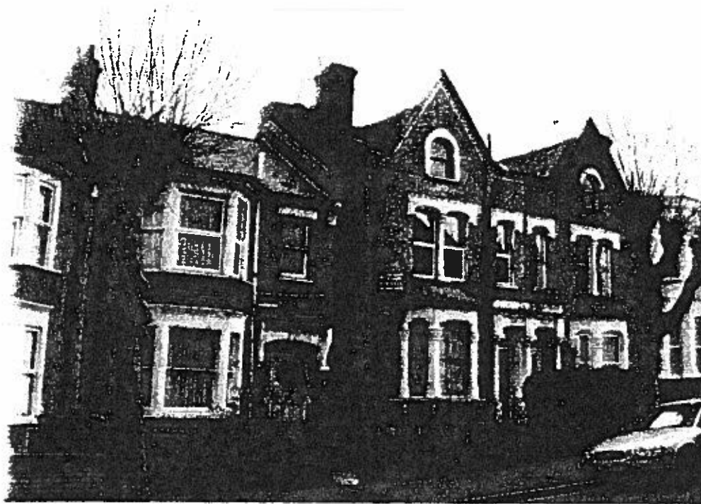
View south along the front of the terrace
