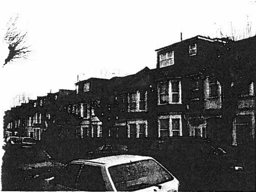
View north along the front of the terrace
