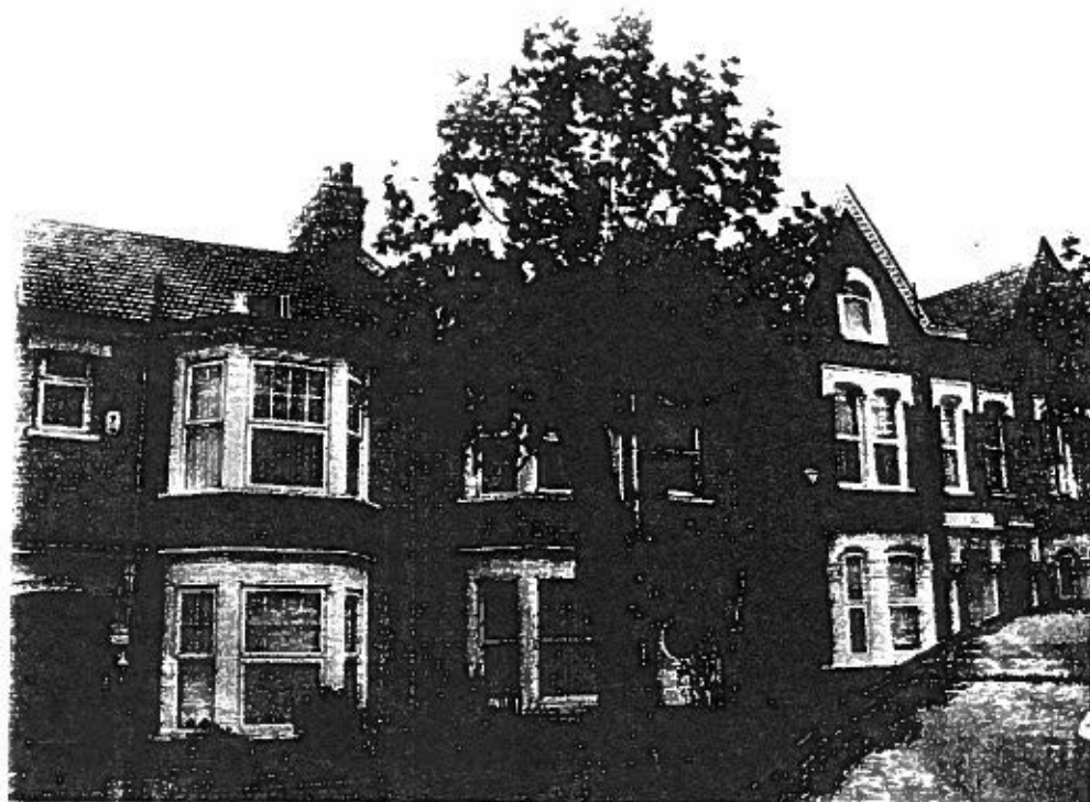
View south along the street
